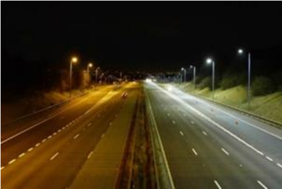
Figure 3: Sodium compared to new LED lighting
